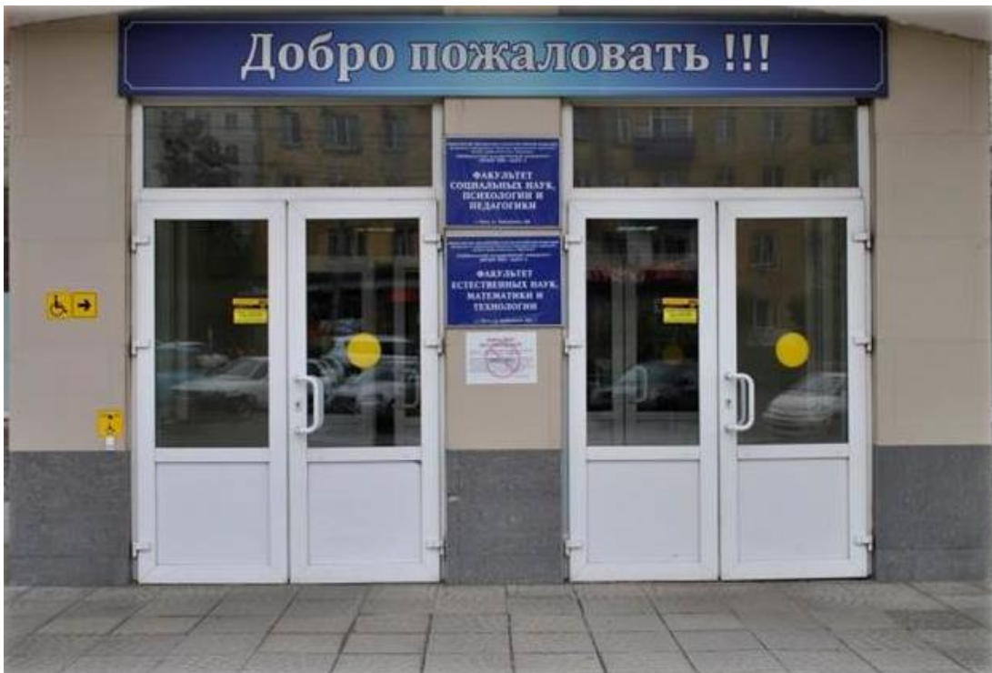
Photo 1 (Author: Sergey Kokhan). The entrance group of the academic building of Trans-Baikal state university. May 2018. Author: Sergey Kokhan
