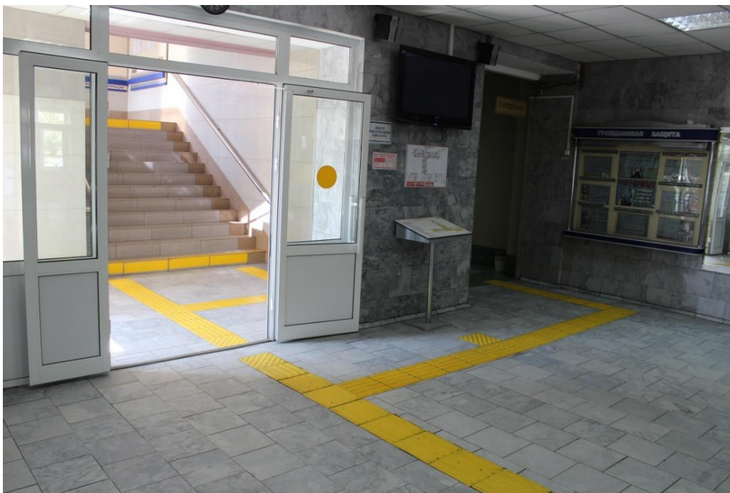
Photo 2 (Author: Sergey Kokhan). Tactile marking of the first floor of Trans-Baikal state university academic building. May 2018. Author: Sergey Kokhan.
